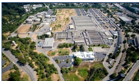
King County South Treatment Plant
