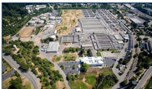
King County South Treatment Plant
