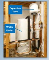
overflows from the main hot water tank and pushes against an air cushion within the expansion tank, causing the air cushion to compress and allowing water to flow in. This alleviates the pressure of thermal expansion by giving the expanded hot water a place to go. The size of the expansion tank depends on the size of your hot water tank, the water pressure, and water temperature.
