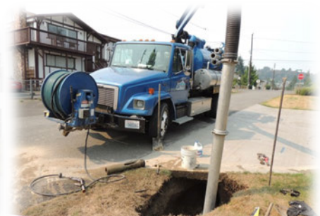
Small Diameter Watermain Replacement
