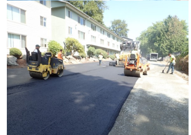
Asphalt paving in progress.
