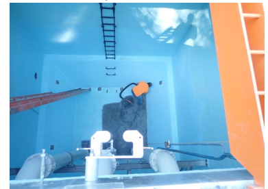
Station wet well primed & coated!
