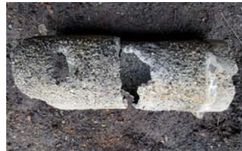
RECENTLY REPAIRED 1950'S ERA 6" SEWER MAIN
